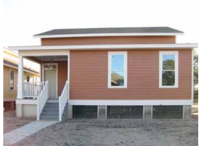
Photograph 7: Elevated and Open Crawlspace —Open pier construction and a trellis couple the crawlspace to the exterior.
