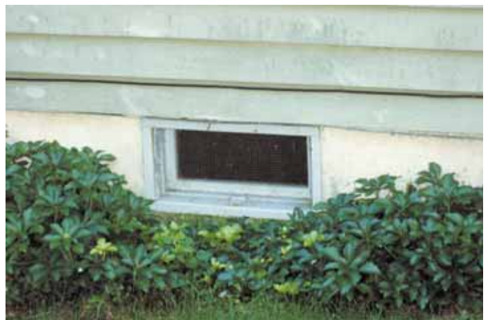
Photograph 3: Ventilation Opening —Crawlspace has plenty of cross ventilation and good drainage.
