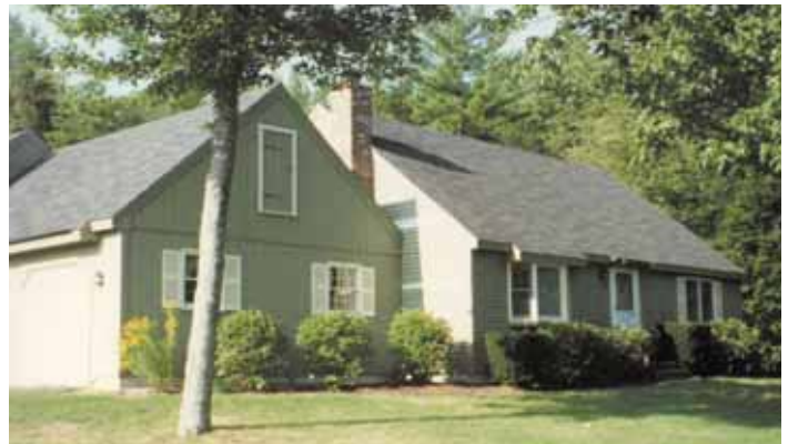
Photograph 2: Nice House Over Icky Crawlspace —This house with the crawlspace problem is in Washington, DC
